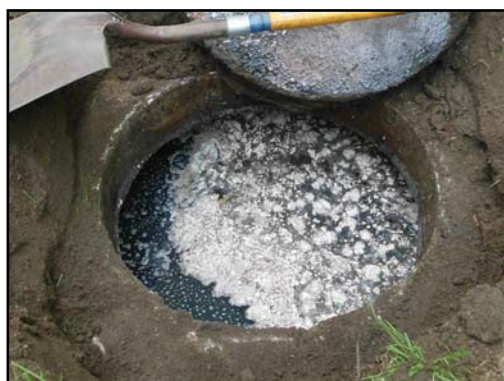
After - septic system recovery, no sludge layer, minimal scum layer
